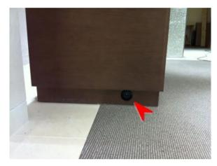
A 52mm diameter hole is required for the rosette to be fitted through the cupboard door, plasterboard wall section, etc. and the extended nozzle section (35mm diameter) passes through a central hole in the rosette.
